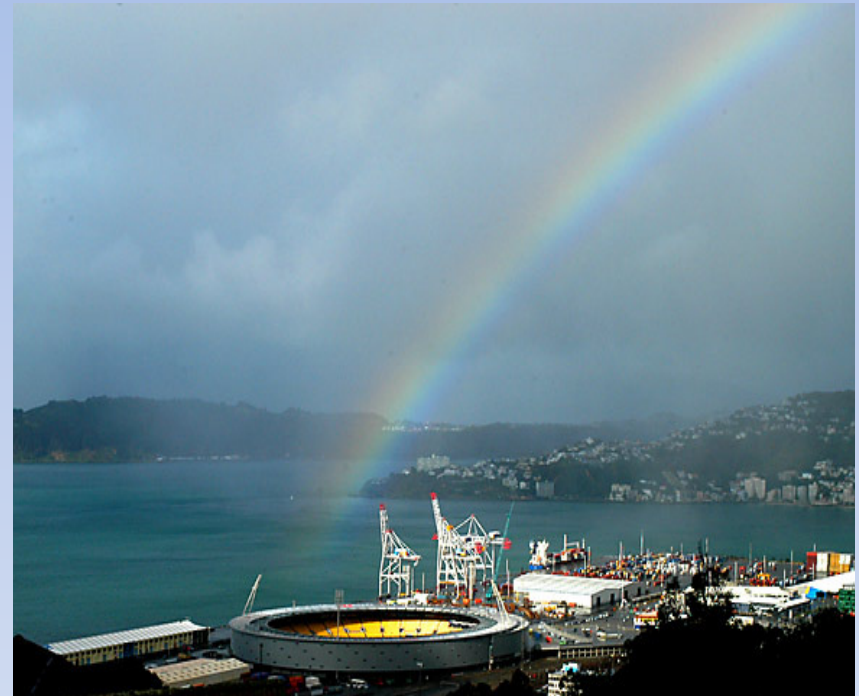
Wellington Stadium 'The Cake tin' home of the Wellington rugby 7's international tournament
